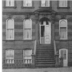
A Tonsil Remedy Is Fitted for a New Century
